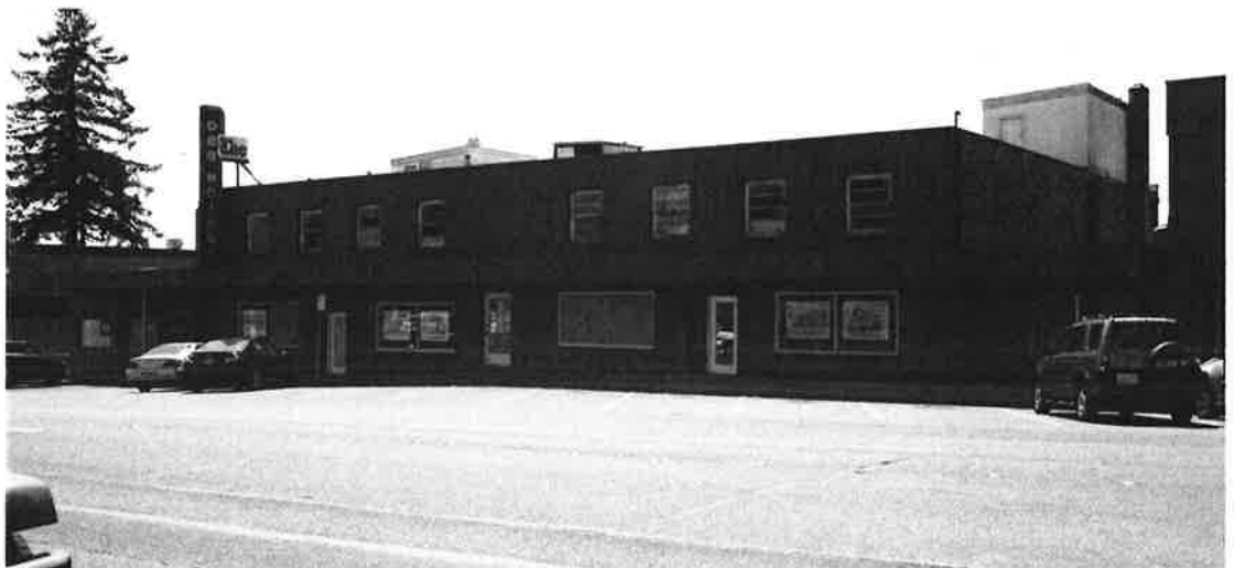
2017 image of the (vacant) Des Moines Theater, 22325-22333 Marine View Dr. South. Photo by Artifacts Consulting, Inc.
